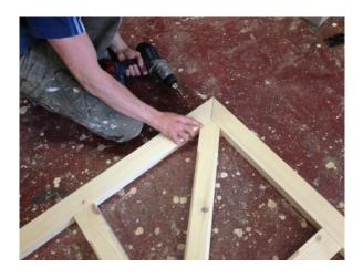
• Now fix the truss to the upright using the fixing supplied through the pre-drilled holes.
