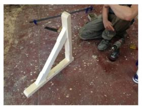
Once the bracket is square fix the remainder of the joints using the screws provided making sure the bracket remands square at all times
