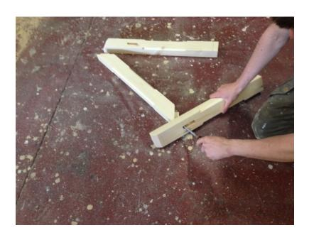
• Dry fit all the joints together to make sure the bracket will go together
