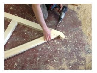
• Now fix the Rafters to the Tie-Bar using the fixing supplied through the pre-drilled holes.
