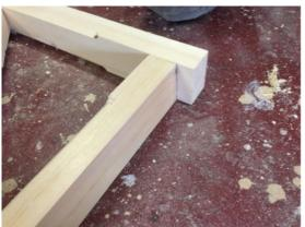
• Ensure all joints can be pulled closed and that the Jamb can be lined up with the manufacture mark.
