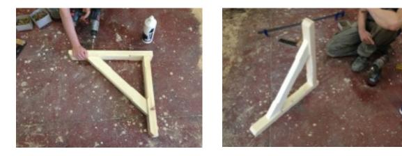
• Once the bracket is square fix the remainder of the joints using the screws provided making sure the bracket remands square at all times
