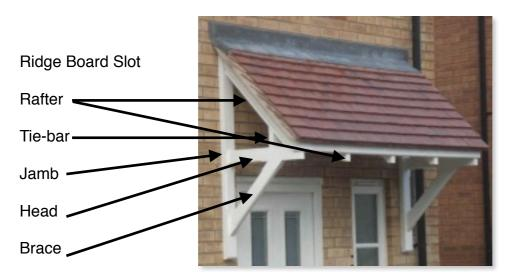
**Step 1 = Assembling the Gallows Bracket Section.**
